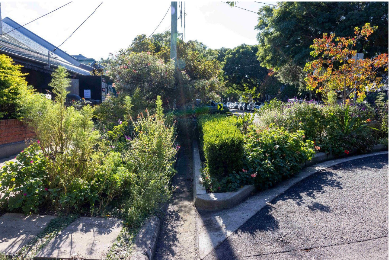
Road Closure garden plantings managed to keep drains and gutters clear. Image: Abril Felman/City of Sydney
